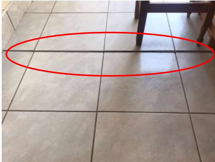
Level difference in bar floor, behind tank
