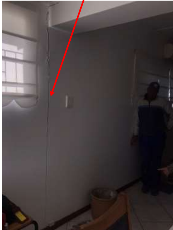
Crack corresponding to crack in second bedroom; View of corner bedroom indicating cracks
