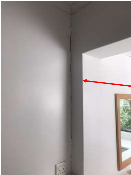
Crack corresponding to crack in second bedroom; View of corner bedroom indicating cracks
