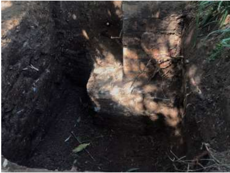
Excavated corner where underpinning is to occur
